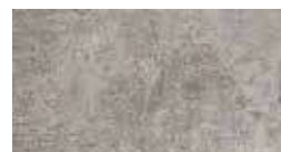
⊗ F8830 ELEMENTAL CONCRETE
